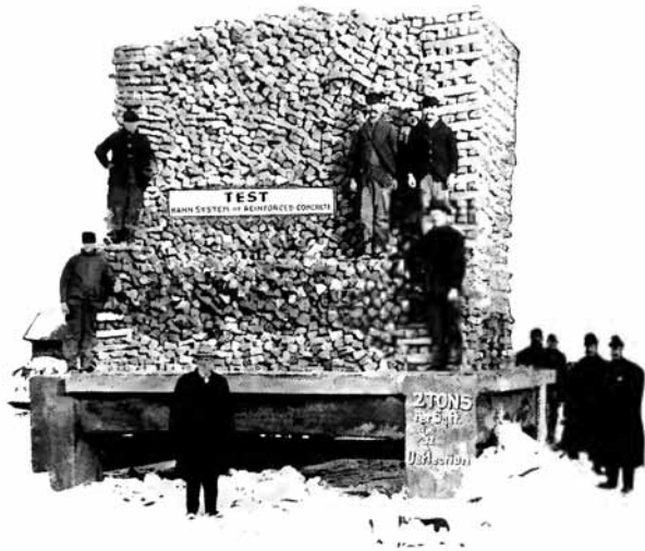
Figure 5: Test panel constructed with the Kahn System loaded to 4,000 psf with iron ingots for the Nichols, Dean and Gregg Warehouse Building in St. Paul, Minnesota (demolished 1990).
